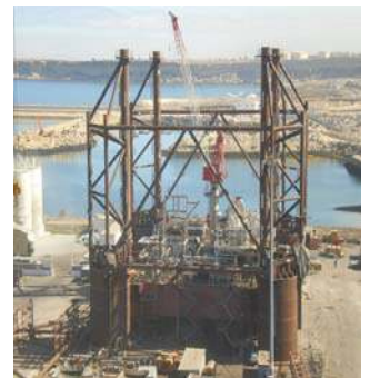
Platform during construction in DLM yard
